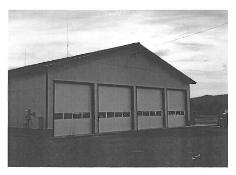
Originally built in the early 60's. Size was approximately the two bay doors to the left in this picture. The station experienced a fire in the late 70's. In 2018, the station underwent a major overhaul to seismically retrofit the building and got much needed upgrades along the way. Items like new bay doors, new siding, roofing, lighting, electrical, bathrooms, floor coverings, exterior doors, upstairs fire exit, and paint were all included in this project.
